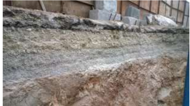
Shows cross section of Pavement-Ameerpet to Punjagutta
